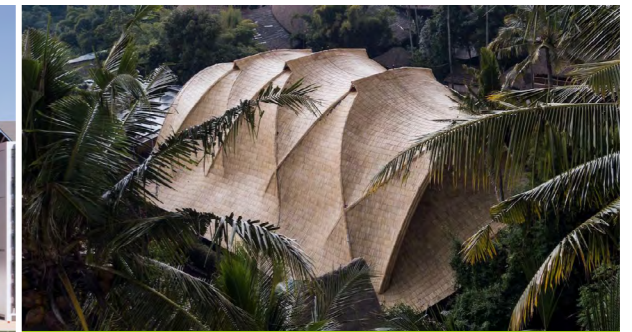
‘The Arc’ of Green School Bali
